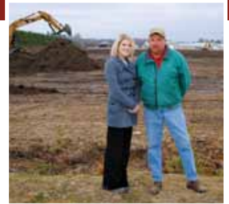
Shannon Bell, Burgaw branch manager (left) and Scrapy Hall with construction beginning in the background on four new poultry houses
